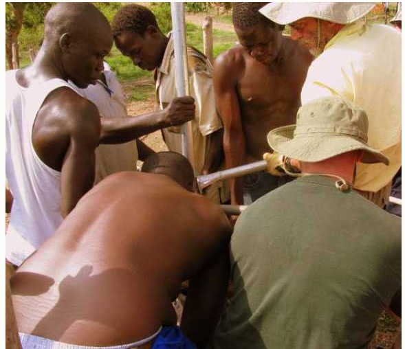
Mike and Dan assist the Sudanese with well repair
